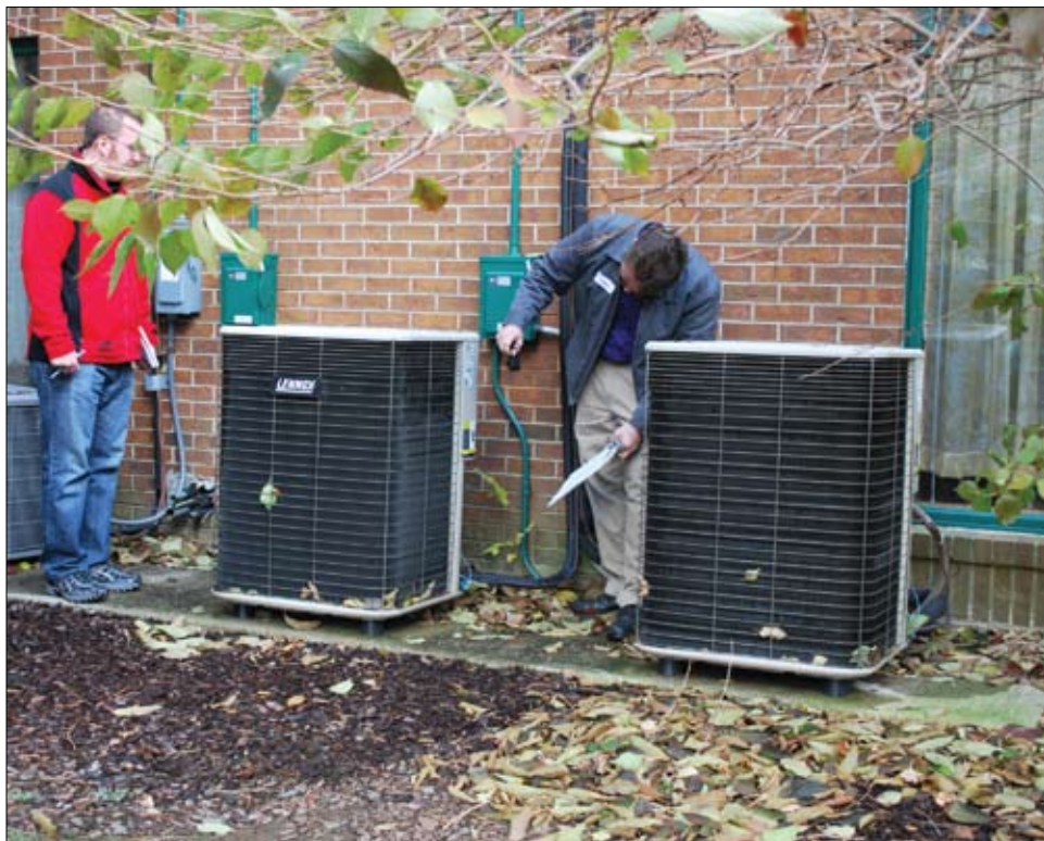
Engineer Lane Freiberger looks at one of the 10 heating/cooling units at KSBA. At left is Engineer Eric DeLodder. The engineers from the Kentucky Pollution Control Center walked through both the inside and outside of KSBA’s Frankfort office to see where energy savings could be found.
